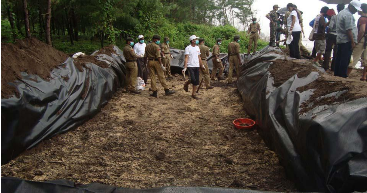
Pit Prepared for the bioremediation with working cadets and TERI
